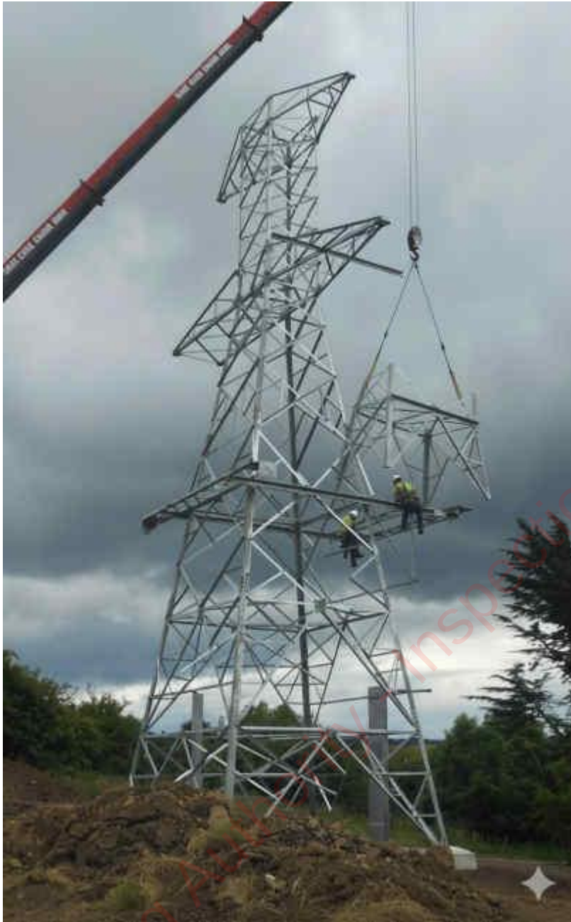
Plate 2-11 End Mast under construction
