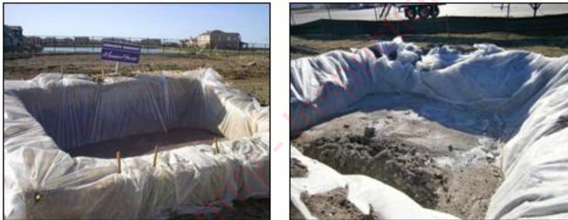
Plate 3-2 Typical concrete wash out areas
