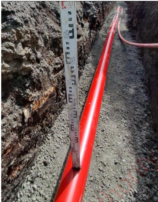
Plate 2-1 Typical Single Cable Trench View
